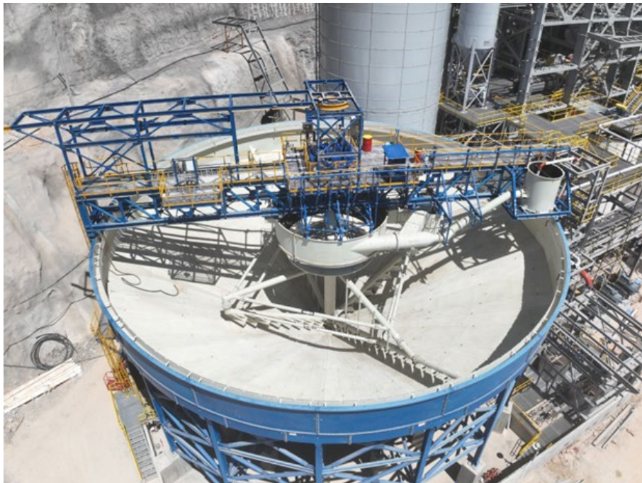
Figure 4: Paste plant thickener ready for water testing.
